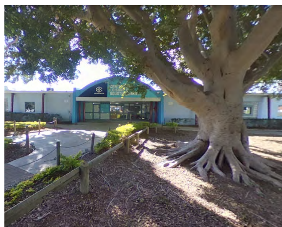
1. existing building entry
