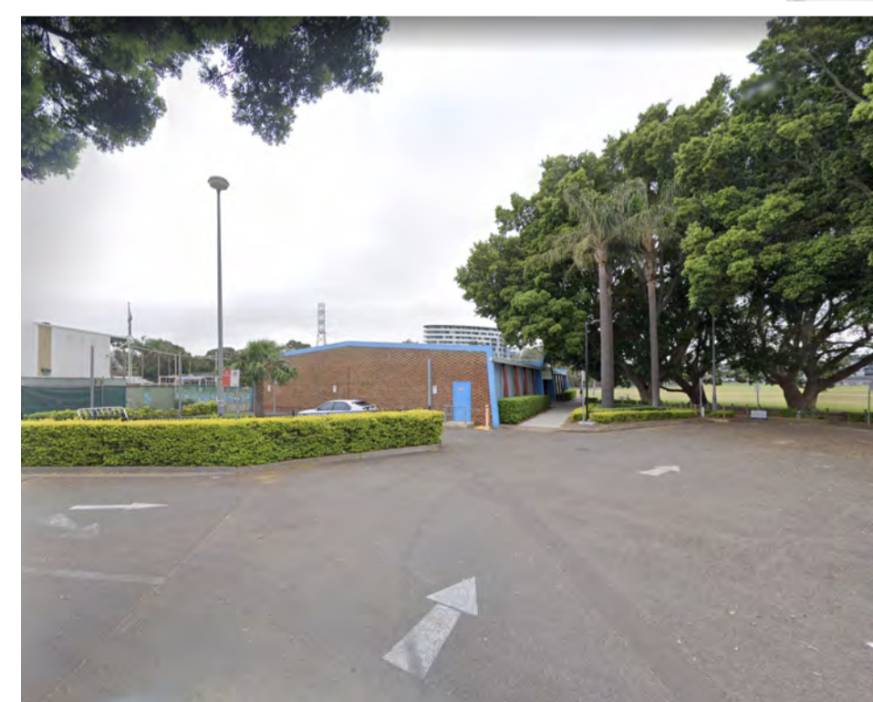
3. view from existing carpark
