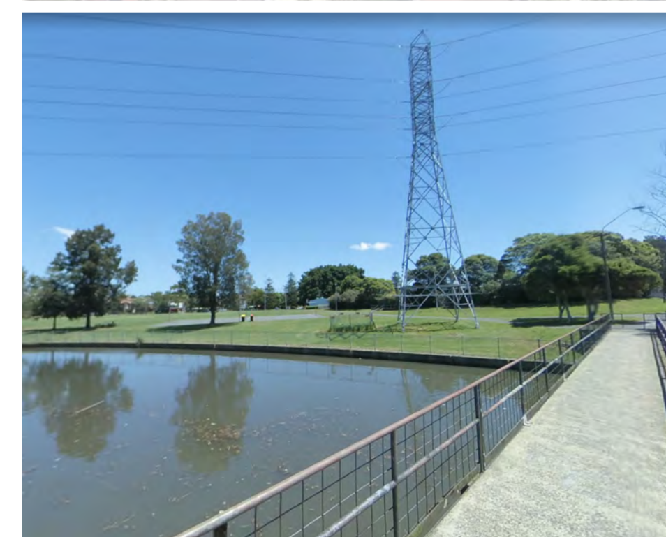
4. view from existing bridge
